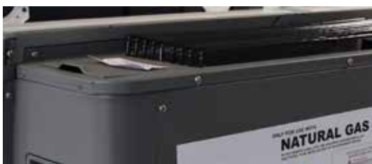
Top vent for natural convection heating
